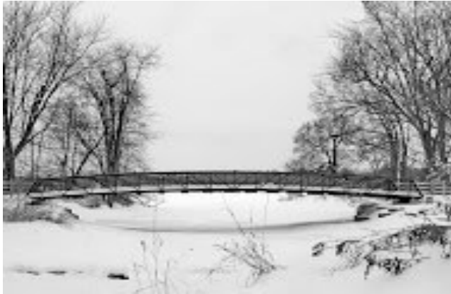
Tollington Bridge At Beavermead © 2016 by Brian Crangle
